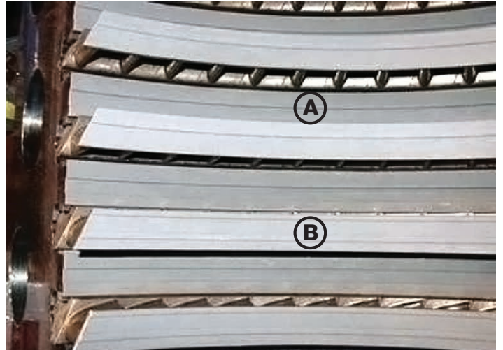
A) Abradable coating applied to the outer steam path seals on the casing. B) Abradable coating applied to the inner steam path seals on the shrouds of the stationary blades.
