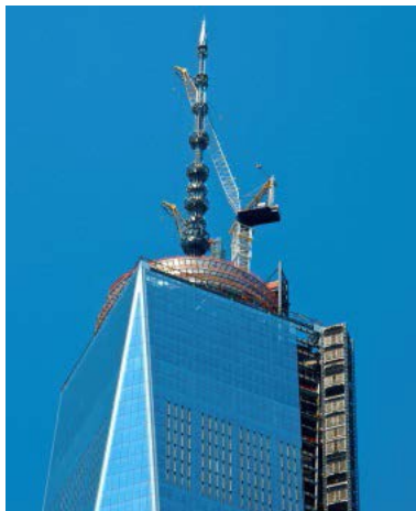
139.6 meters, 680 metric tonnes: The spire of One World Trade Center
